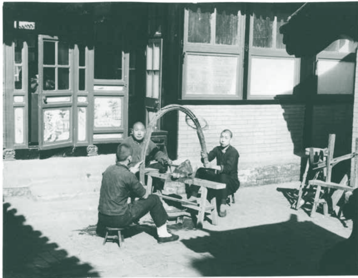
S. Howard Hansford CHINESE JADE CARVING, (Lund Humphries) Pl. IV b Original photograph taken by the author in Peking Apprentices sawing a block of jade with a wire saw carrying abrasive "sand" (carborundum) mixed with water.
